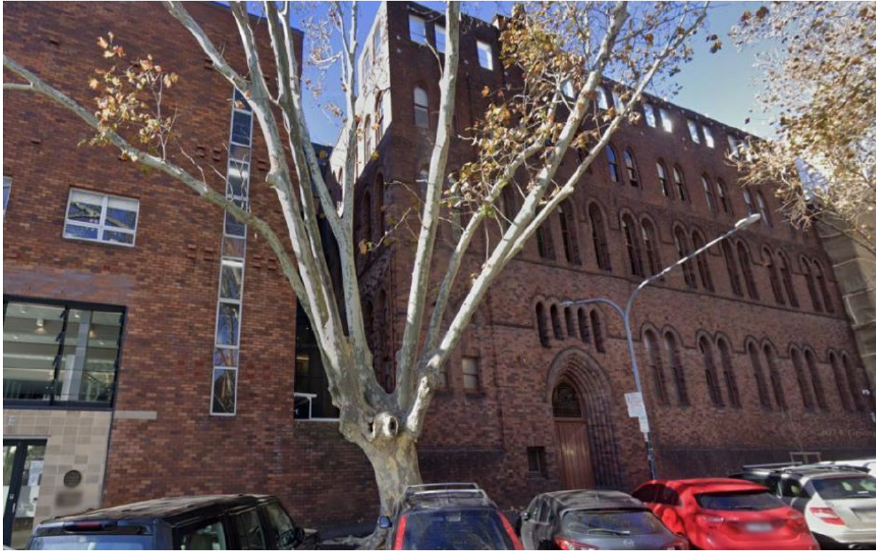
Vincentia building & Mary Aikenhead building on Victoria Street
